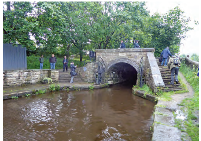
Dingle end portal showing extension added when the double-track railway tunnel was added. Photo Bob Clary
